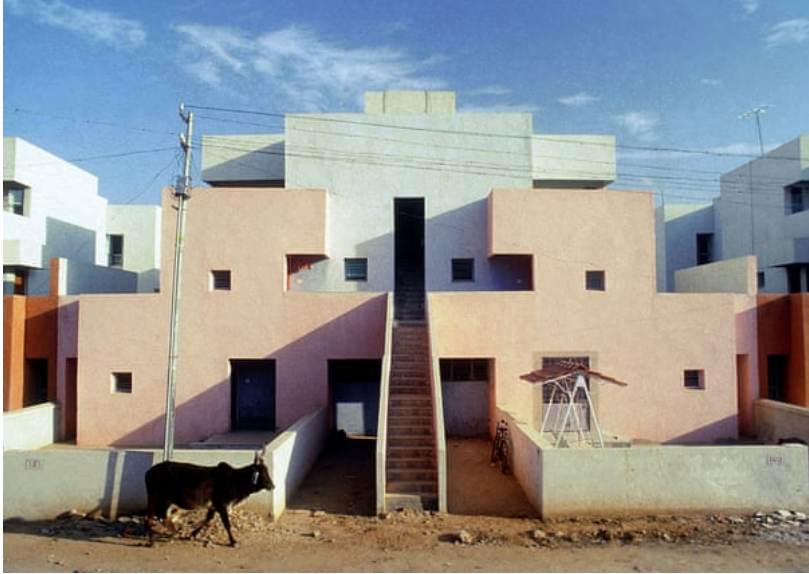
Housing for a life insurance corporation, Ahmedabad, India, designed by Balkrishna Doshi Photograph: Courtesy of VSF
