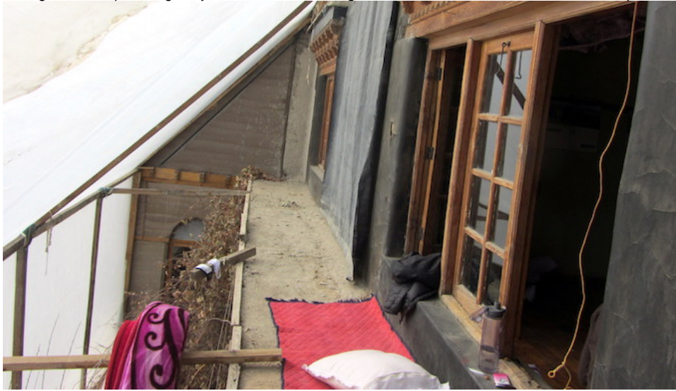
The plastic sheet traps heat and prevents chilly winds from entering during winters. In summers, this is rolled up to let in fresh air (Photo by Nivedita Khandekar)
