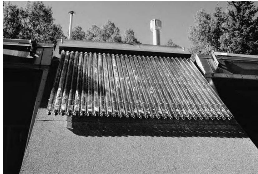
*8.12: One of the newest and most efficient solar hot-water systems made by Thermomax, this rooftop collector heats water for domestic uses, even heating the home.*
