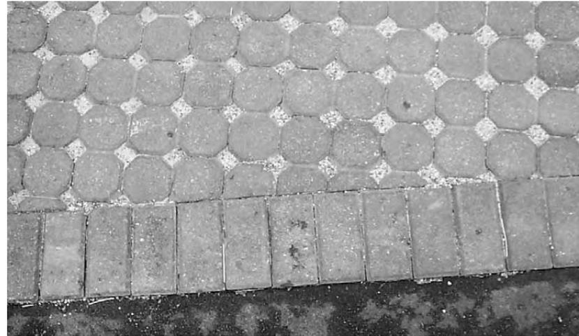
*6.3: Porous pavers like these let moisture seep into the ground, reducing surface runoff, flooding, and nonpoint source water pollution. Porous pavers and other similar strategies reduce heat-absorbing pavement, making homes much cooler in the summer while reducing utility bills. Credit: Turfstone Company.*
