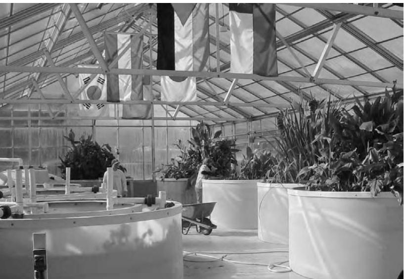
*9.2: The Living Machine is a greenhouse-contained biological waste treatment facility that uses natural methods rather than harmful chemicals to recycle human waste.*
