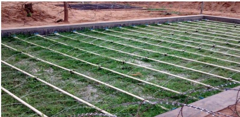
The sewage is automatically distributed on the Bioreactor and converts to grass and clean water. It comprises a 1.5 mtr deep tank with bio-media
