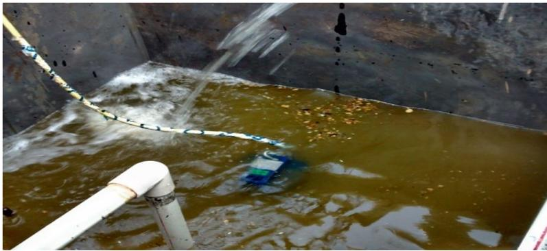
The fresh sewage is automatically mixed and pumped onto a Bioreactor. 10% of treated clean water is recycled here to initiate the treatment.
