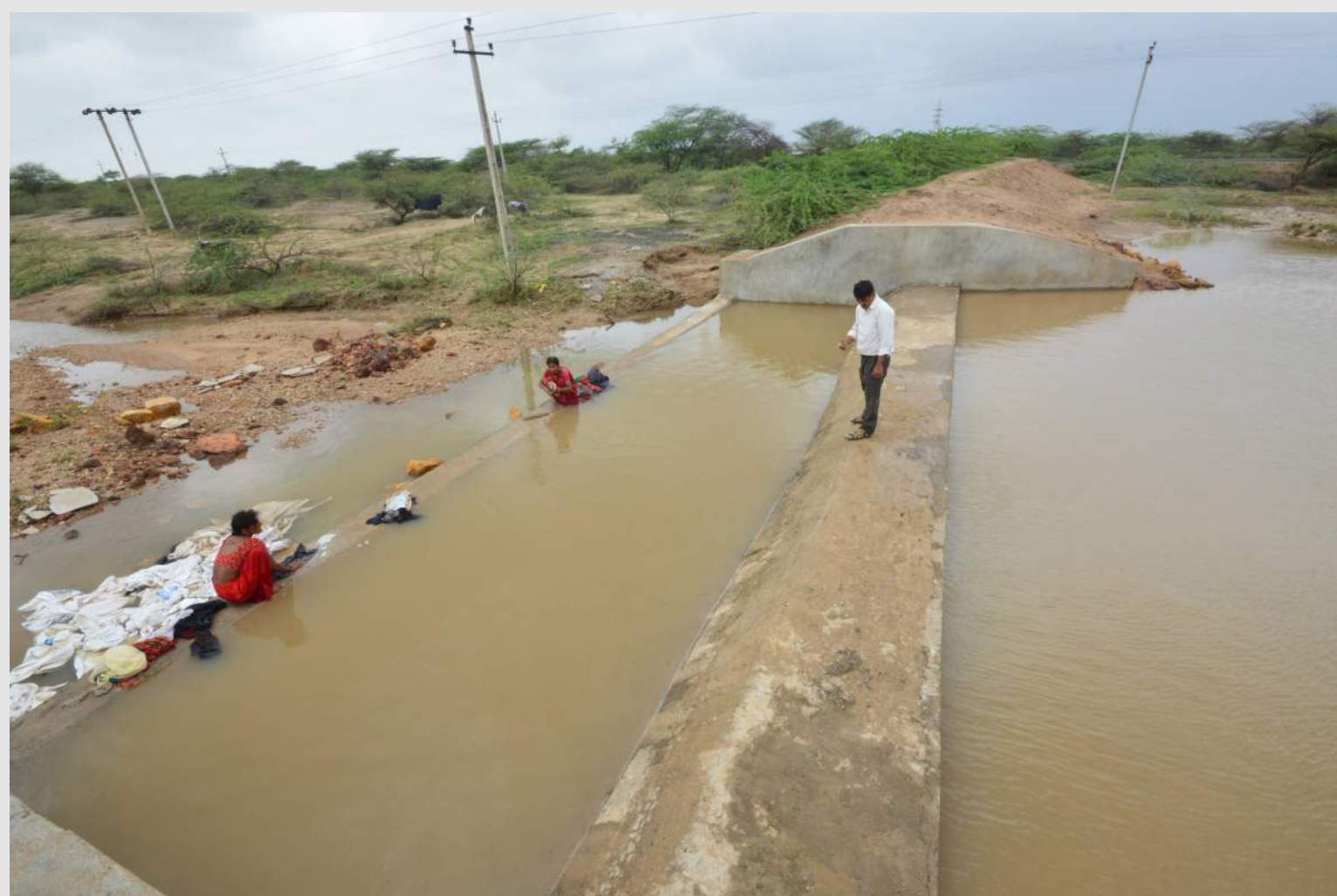
Left: Small check-dams to prevent water run-off in Abdasa, Kachchh.
