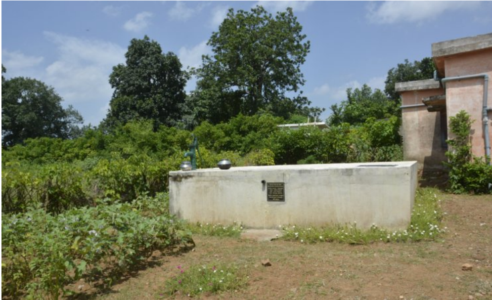
Rainwater harvesting tank at Madiya Kachar village school
