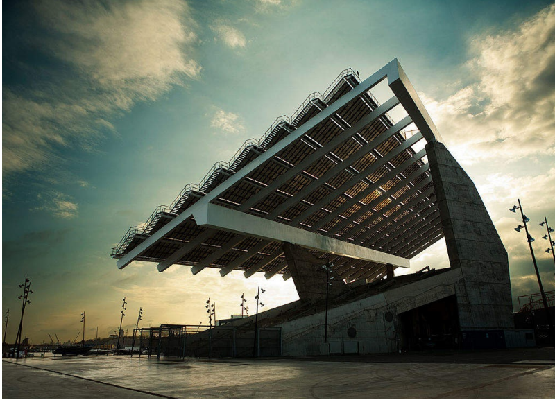
KOZHIKODE: The Kerala State Electricity Board Limited's Soura Roof
